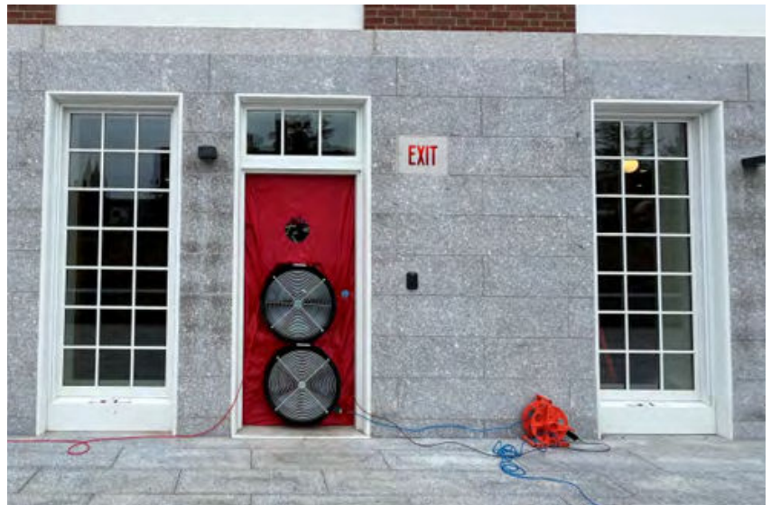
Installed blower door for whole building air leakage testing.
