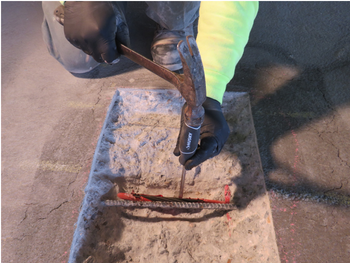
Screwdriver penetration testing of unbonded post-tensioning.
