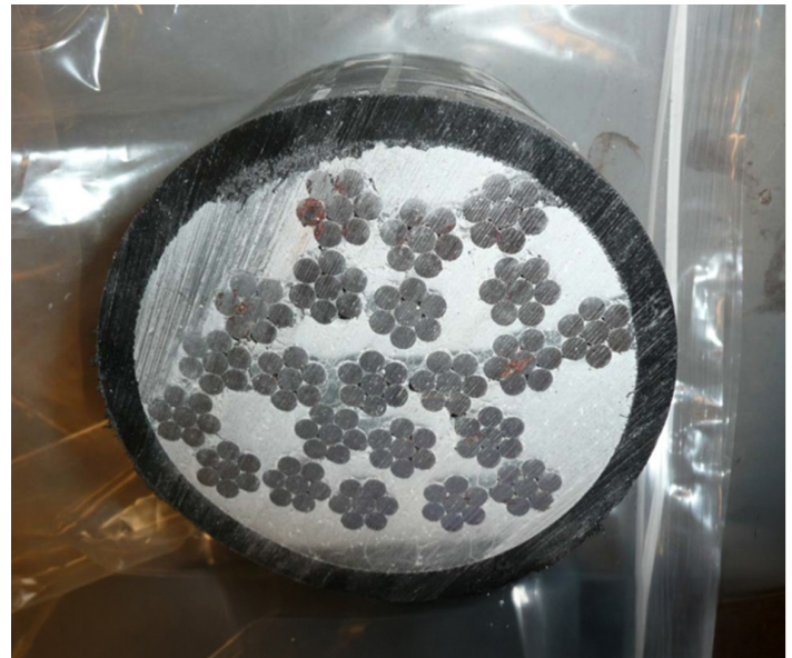
Exploratory opening to examine strands and grouting in bonded post-tensioning.
