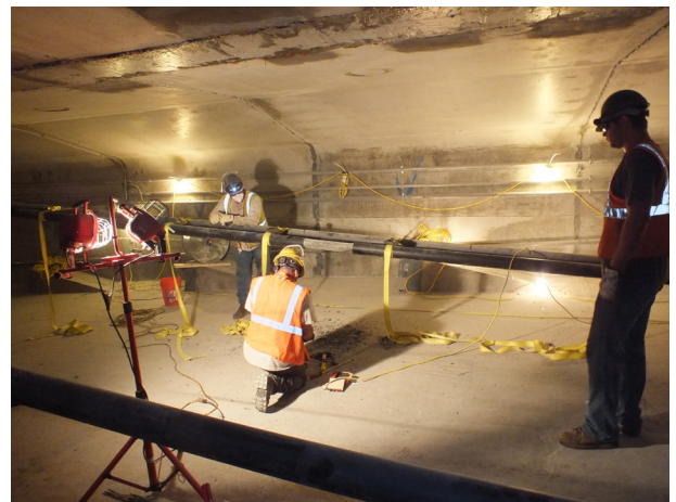
Bonded post-tensioning used for a bridge setting.
