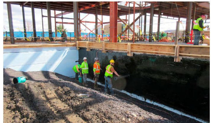
Below-grade waterproofing review (Pennsylvania State University, Palmer Museum of Art, University Park, PA).
