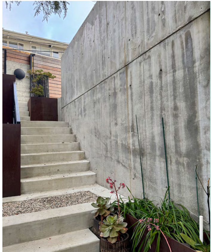
Noncombustible exterior walls can help withstand the risks posed by wildfires in WUI areas.
