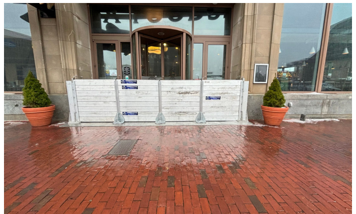
Flood shields outside retail space near Boston Harbor.
