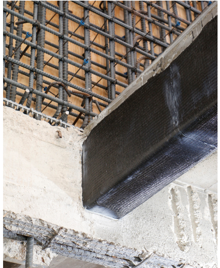
FRP-wrapped beam and rebar for new concrete wall above.
