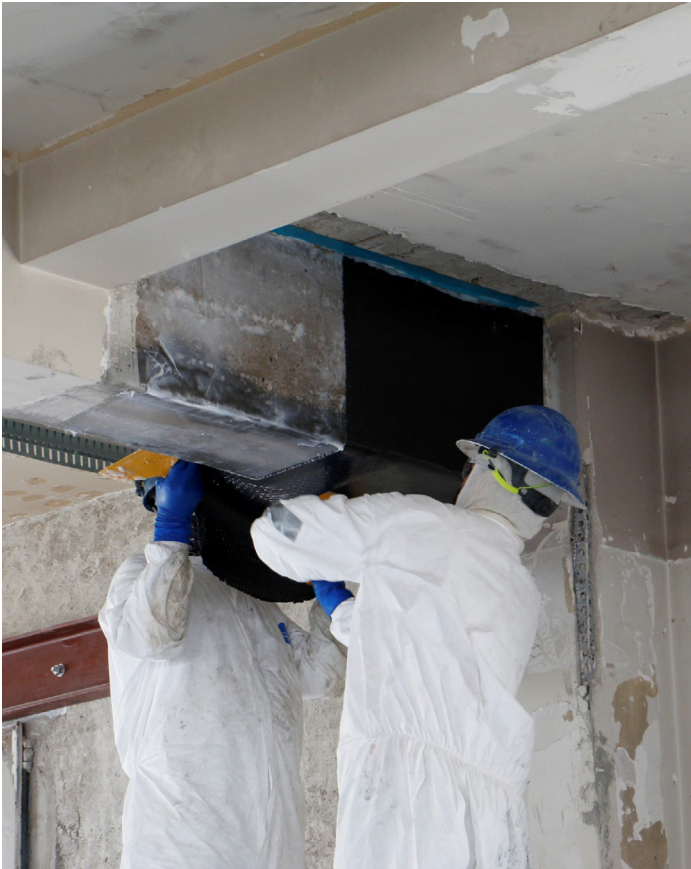
Wrapping a beam in FRP.
