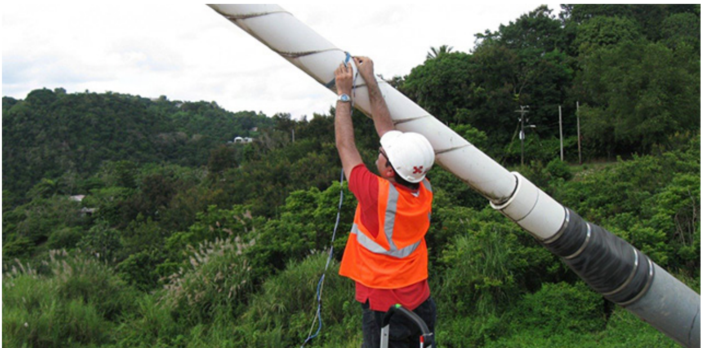
Connecting accelerometer to a stay cable for tension and damping measurement
