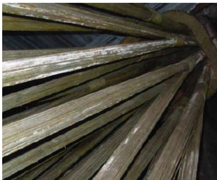
Wire strands at the main cable anchorage
