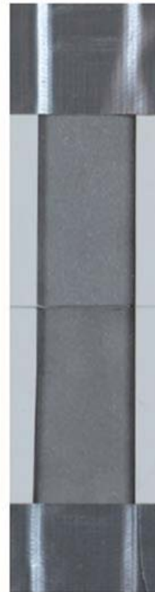
Sandblasting to SSPC SP-5 white finish
