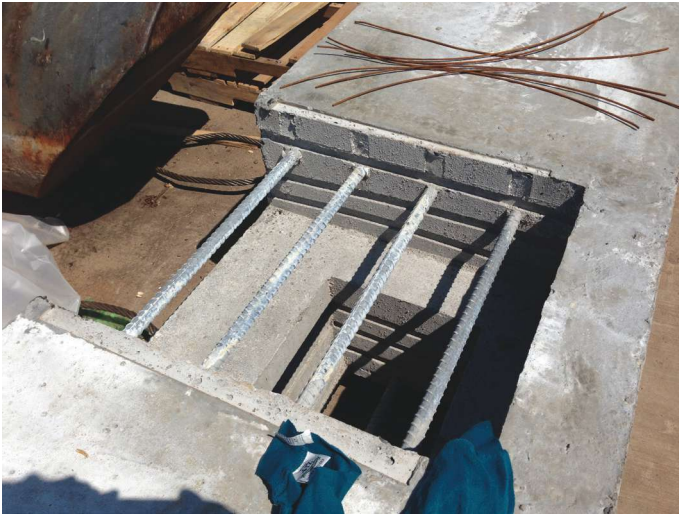
Fig. 11: Pile-beam connection prior to assembly
