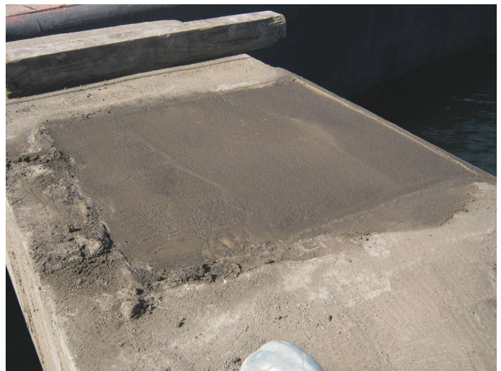
Fig. 13: Pile-beam connection after grouting with rapid-strength-gain repair mortar
