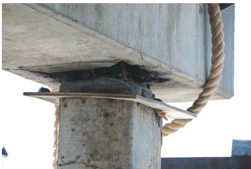
Fig. 6: View of lifted beam at west extension of pier
