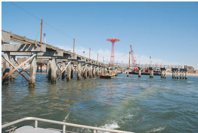
Fig. 2: Overview of pier construction (some existing wood decking and framing remains)
