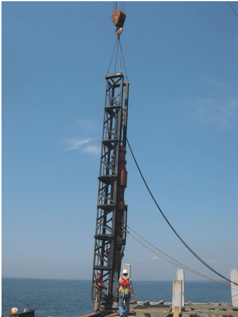
Fig. 10: Overview of driving new replacement pile
