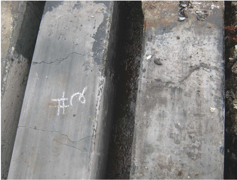
Fig. 9: View of damage to affected piles, after removal, below mudline
