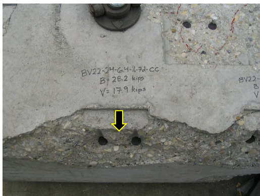
Figure 8 – Test BV22-24-6.4-1/2-7d-CC with a bearing stress of 0.2f'_c .
