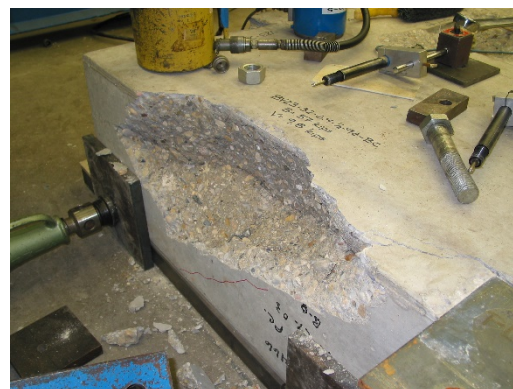
(b) Breakout concrete removed showing the vertical rear crack surface to a depth lower than the studs. The studs did not intersect the crack failure surface.
