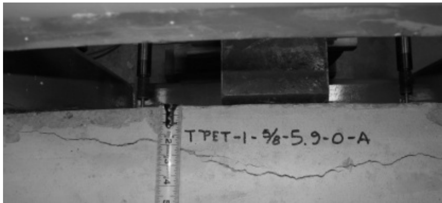
Figure 6: Single stud concrete failure
