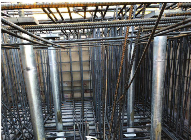
Steel trumpet casings over mat foundation tie-downs on top of a mud slab.
