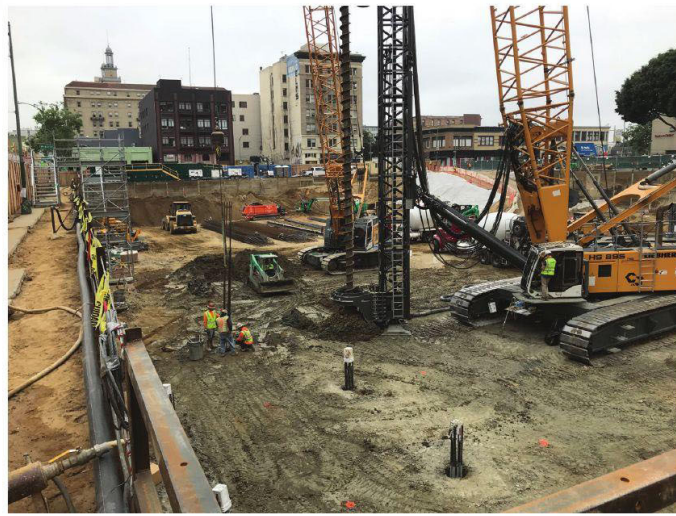
Hollow-stem auger cast drilling in progress.
