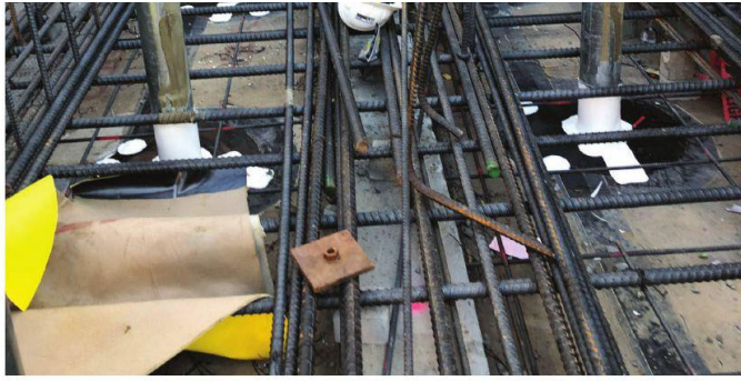
Waterproofing at base of steel truss within a large mat foundation reinforcing cage.
