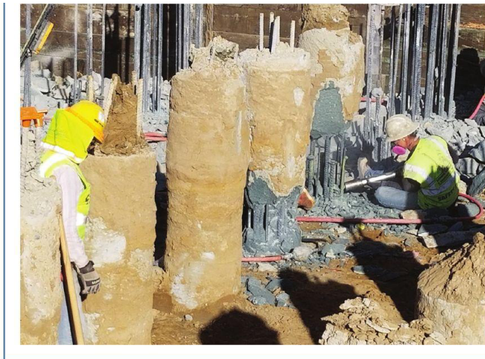
Auger-cast piles for a mat foundation chipped down as excavation progresses.
