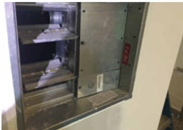
Example of a Fire/Smoke Damper SGH photo
