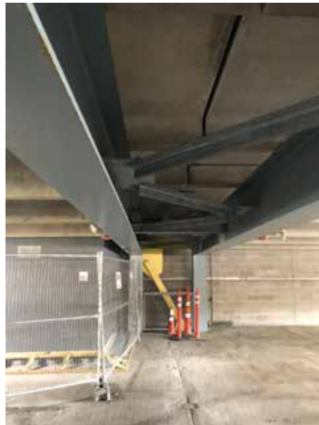
Figure 3. Supplemental horizontal steel bracing to the restore diaphragm connection to LLRS.
