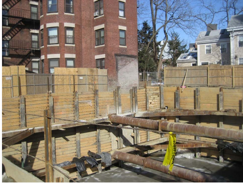
Fig. 2 – Proximity of excavation to existing adjacent structure.
