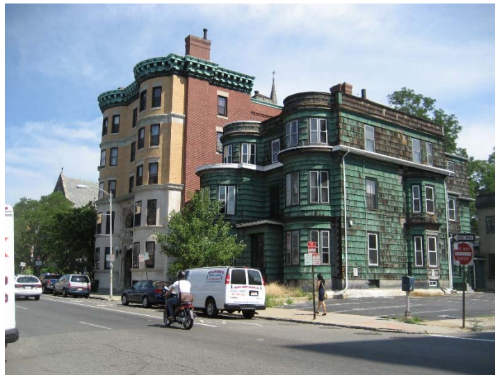
Fig. 1 – Building to be demolished on right, adjacent structure to the left.
