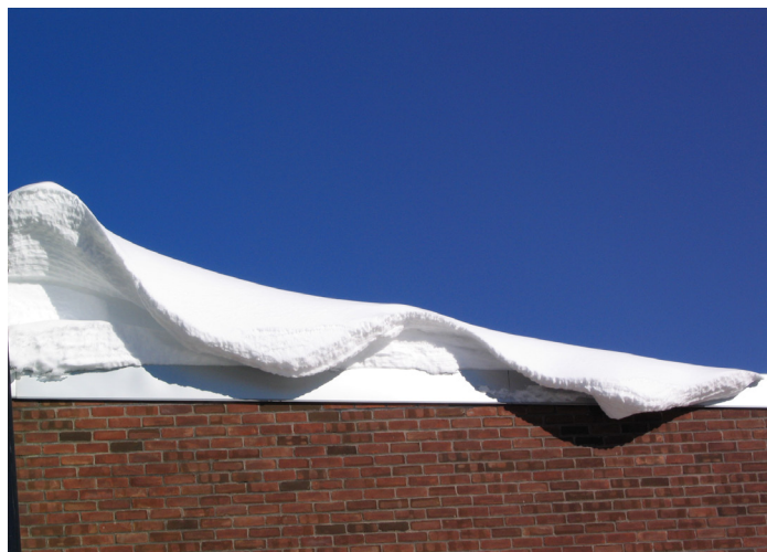
Snow drift resulting in unequal distribution of snow loads
