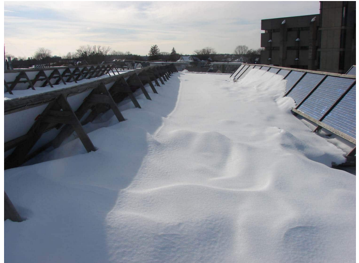
Snow on roof structure
