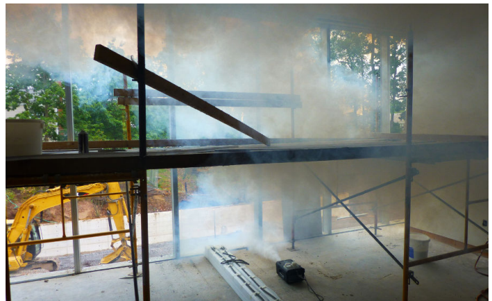
Air leakage testing
