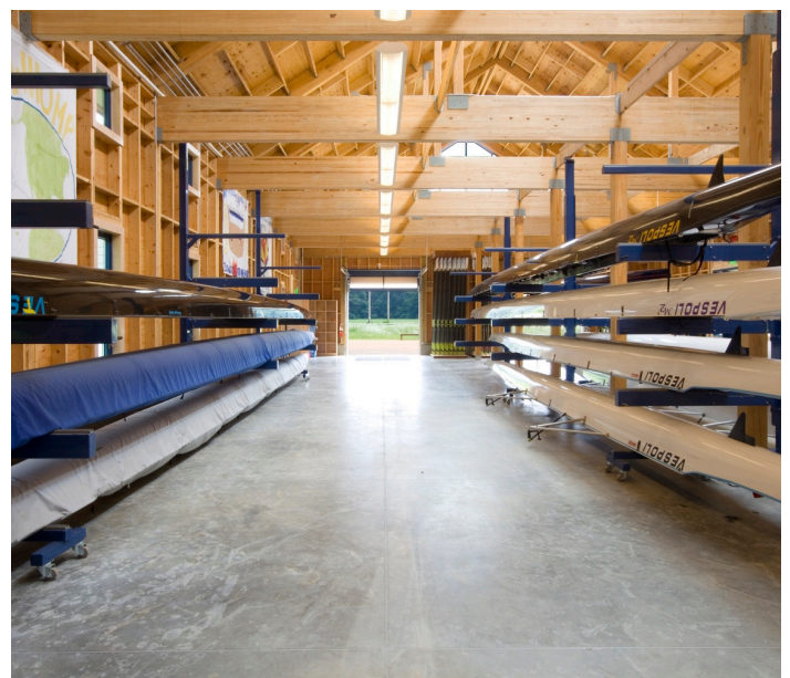
Boathouse using wet floodproofing design
