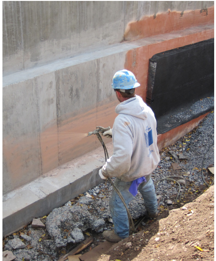
Spray-applied, below-grade waterproofing application
