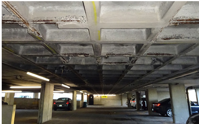
Parking structures, 1279 Pennsylvania Avenue, Brooklyn, NY
