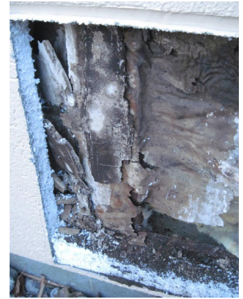
Barrier EIFS at wall base (left). Despite its clean, recently painted appearance, sampling at this location reveals substantial water damage to the wall sheathing and steel framing behind (right).
