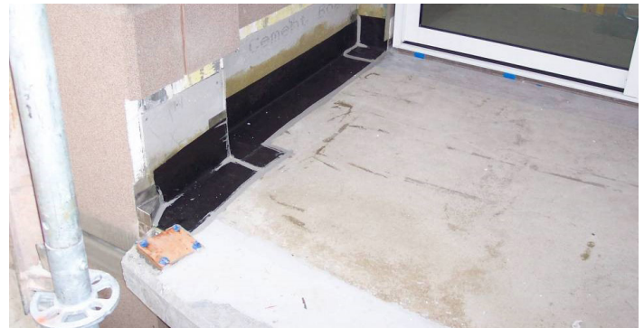
Balcony transition to EIFS wall retrofit with watertight flashing.
