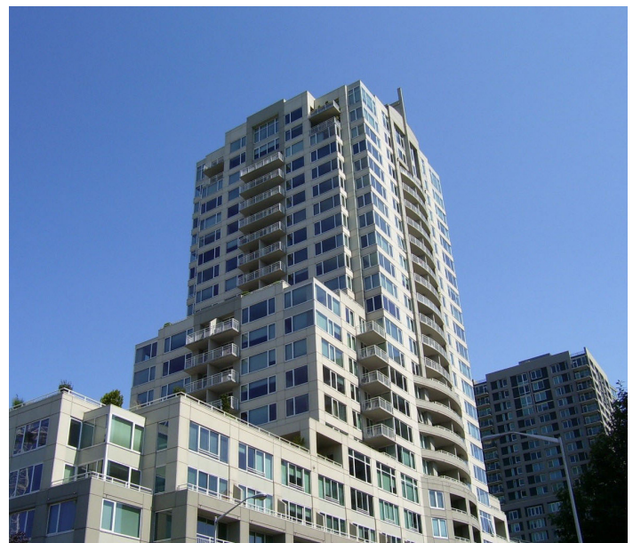
High-rise, barrier EIFS-clad condominium building retrofit with new windows, sealants, flashings, and waterproofing systems at critical transitions to successfully correct water intrusion issues.
