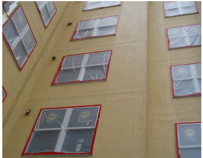
Construction of a drained EIFS system. The wall is covered with an air and water resistive barrier integrated with windows, making the wall weathertight prior to applying the EIFS.
