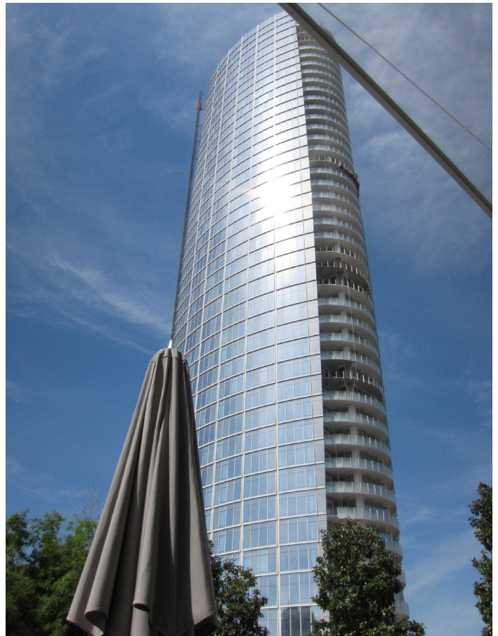
Unanticipated reflections from an adjacent building. Photo by David Norris.
