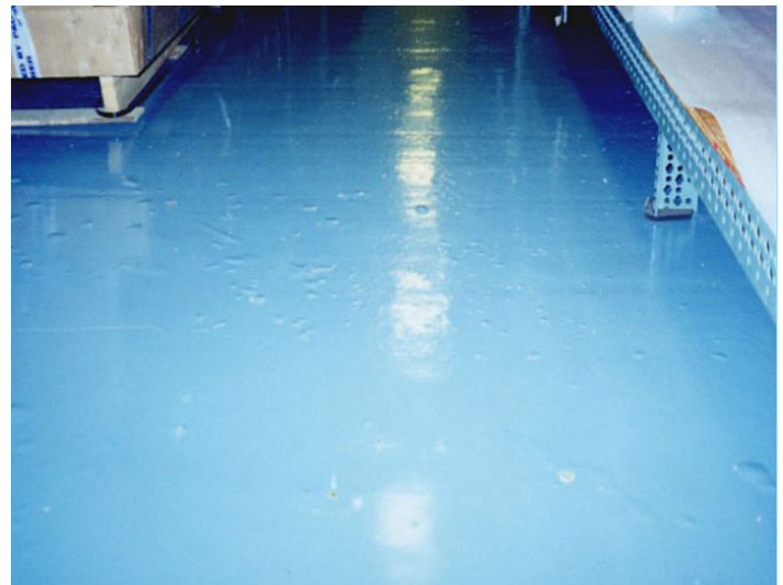
Blistered epoxy floor coating
