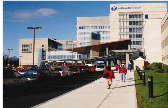
University of Massachusetts Medical Center, Worcester, MA - investigation of stone cladding and modernization of nine-story building.
