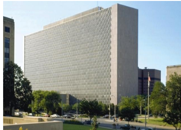
Richard Bolling Federal Building, Kansas City, MO - modernization of a circa 1960s, eighteen-story federal office building.
